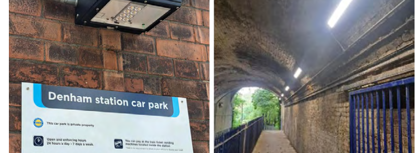
Lighting at Denham station ^
